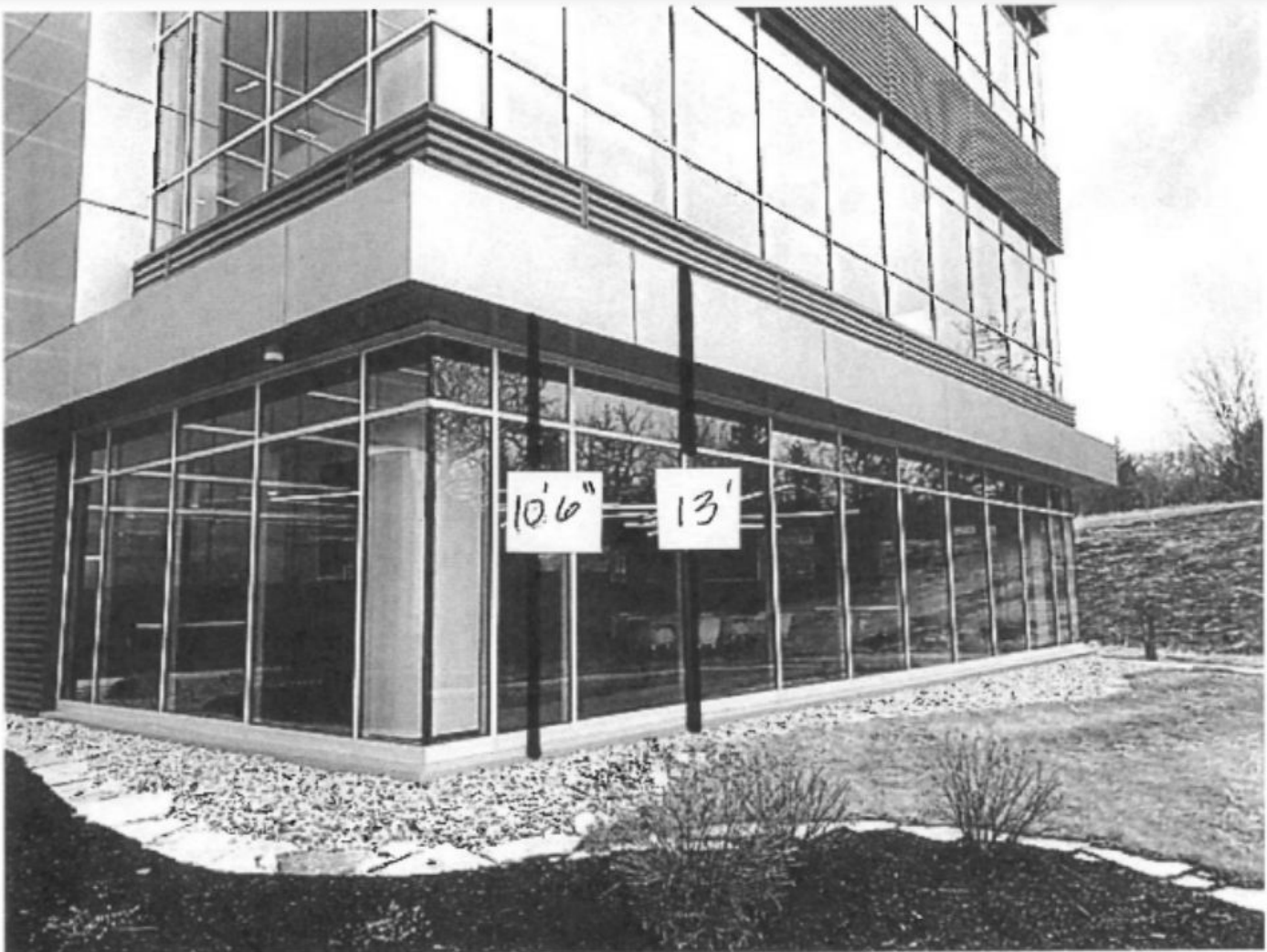
Figure 4- Ground Level Angle Showing First Floor Window Height Dimensions
