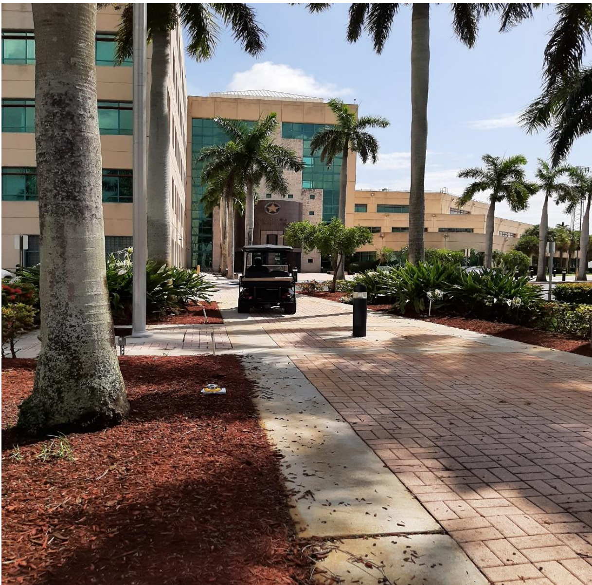
View of pedestrian walkway looking towards the BSO's Public Safety Complex from Broward Boulevard
